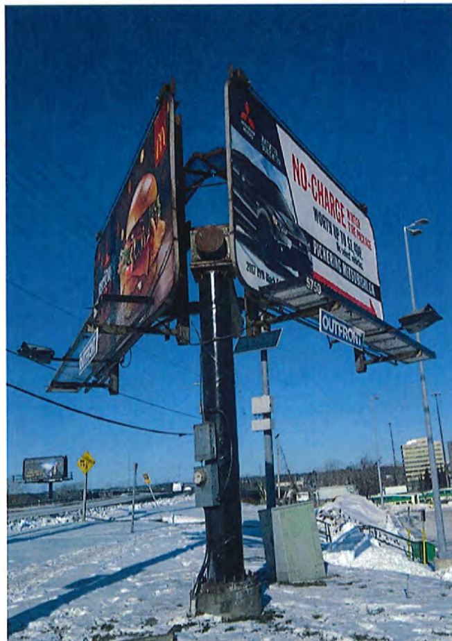
Conversion of existing static sign – Bayly Street east of Liverpool Road
