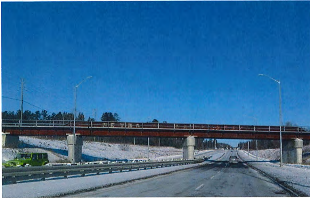
CN Bridge – Brock Road south of Taunton Road – Conversion to static/digital signage on fascia
