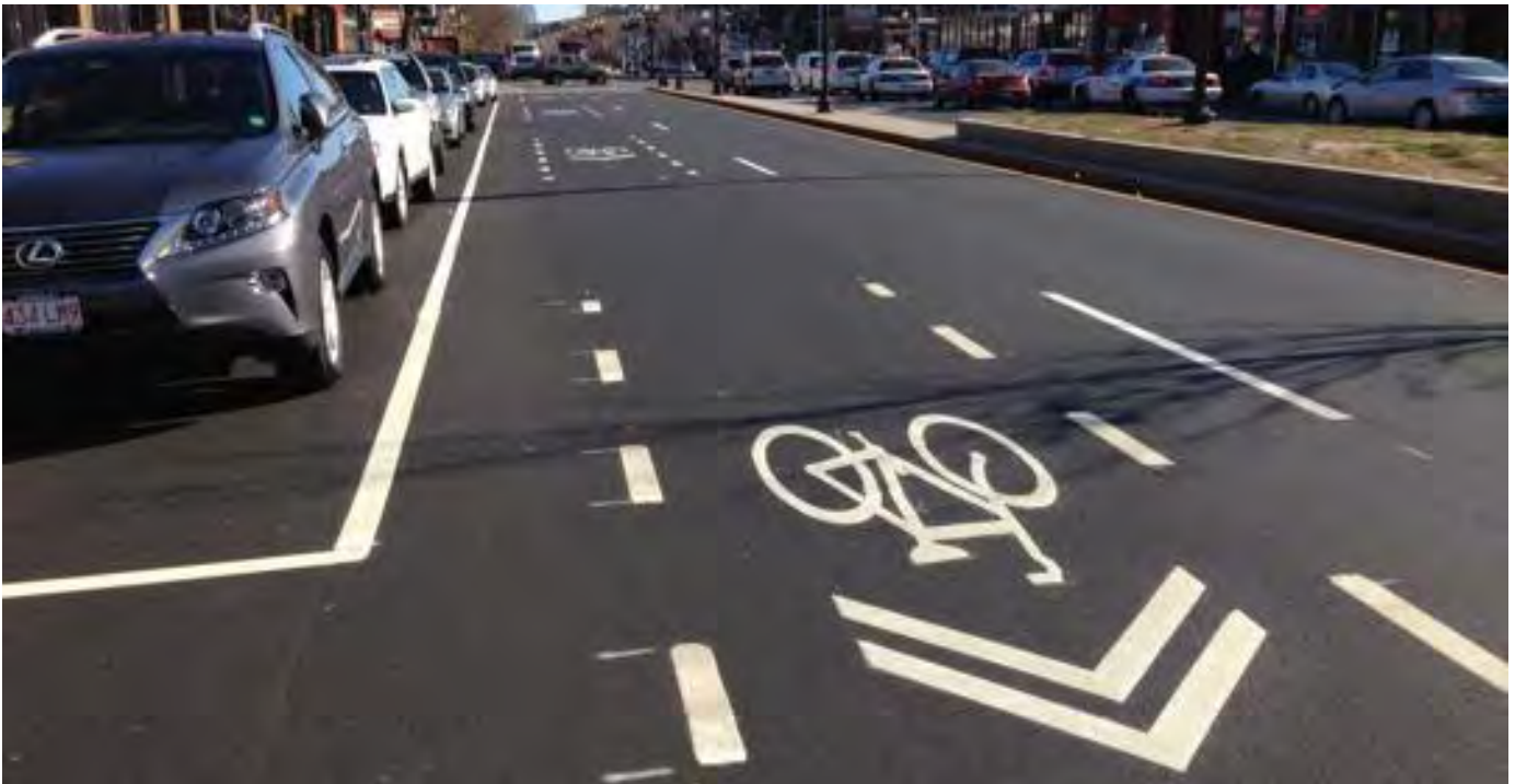
Figure 80. Shared Cycling Facility on Brighton Ave, Boston, USA (photo credits: Boston Globe)
