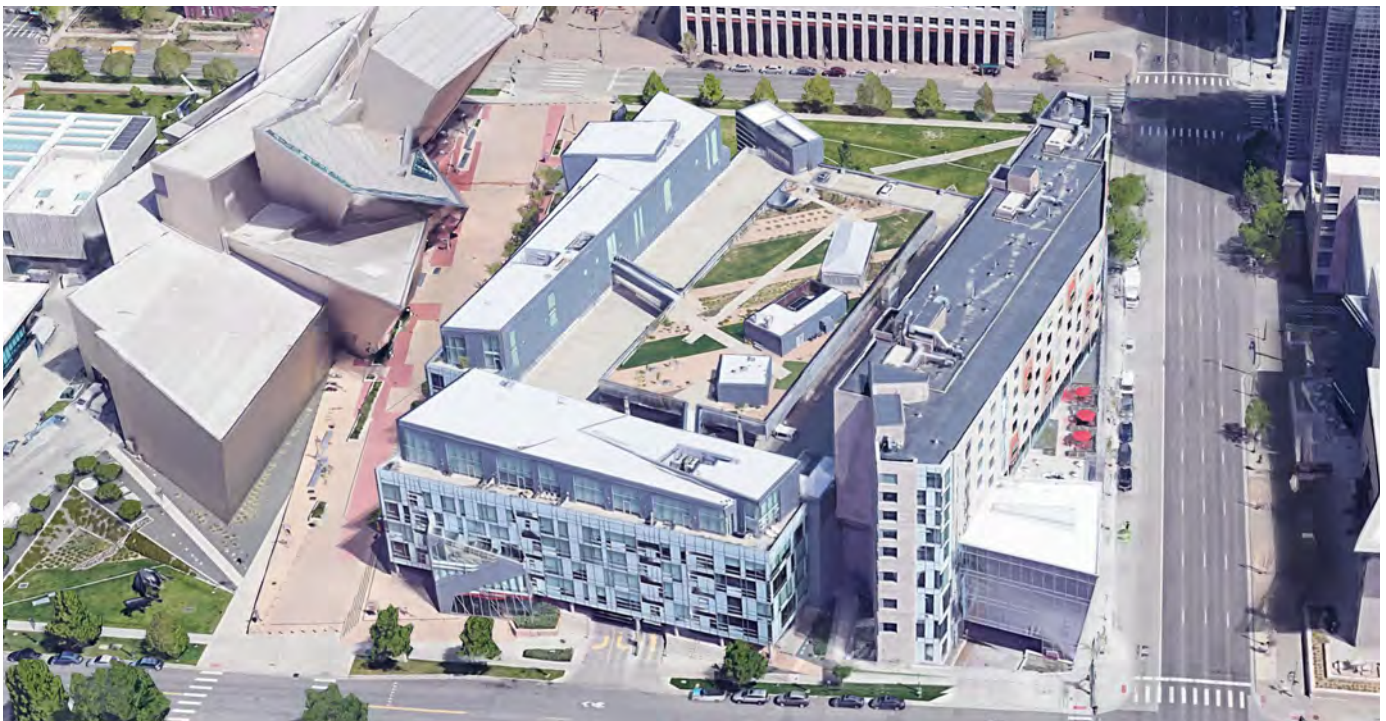
Figure 25. Denver Museum Residence, a 'Texas Doughnut' featuring buildings wrapped around interior parking structure, Denver, USA (photo credits: Google Earth)
