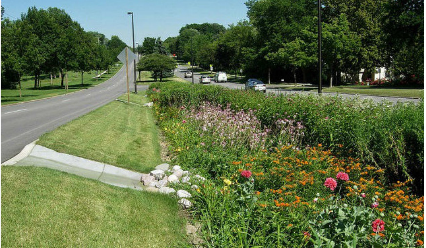
Figure 26. Bioswale system within a median, Detroit, USA (photo credits: Aaron Volkening via Flickr)
