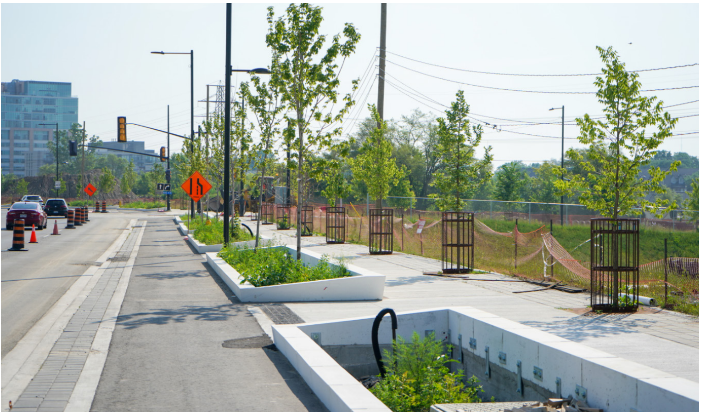
Figure 37. SvN Landscape Six Points Interchange, Toronto, Canada (Image Credits: SvN)
