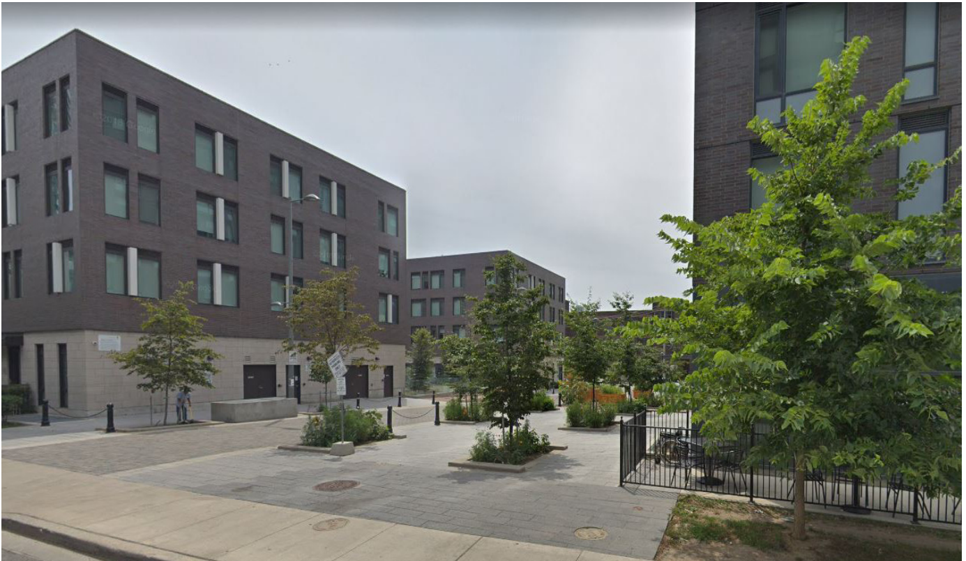
Figure 50. Lower River Street in the West Donlands, Toronto, Canada (photo credits: Google Maps)
