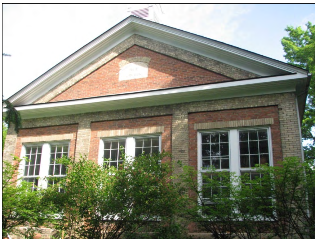
Figure 13: Front elevation with double windows and dichromatic brickwork (AB, 2015)
