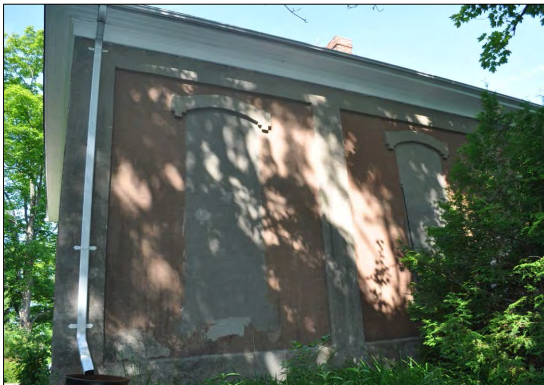
Figure 14: East (side) elevation, with windows filled in and painted stucco covering the exterior brick (CU, 2015)
