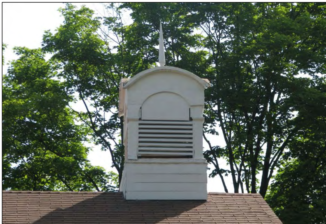
Figure 11: Wooden cupola on the ridge line (AB, 2015)
