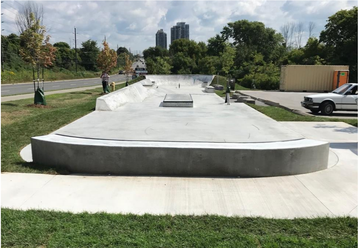
1 West Shore Skate Park View from West Shore Community Centre
