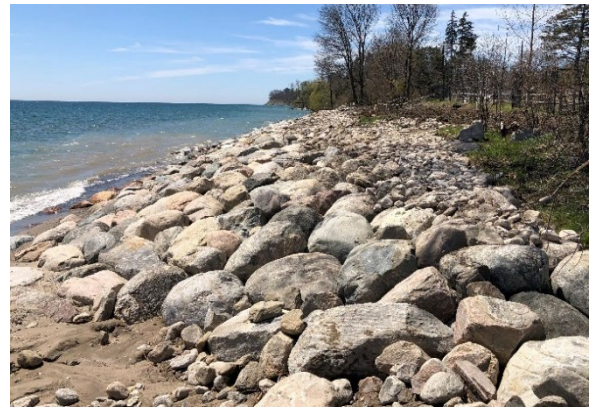
Beachfront shoreline restoration at Rotary Frenchman's Bay West Park
