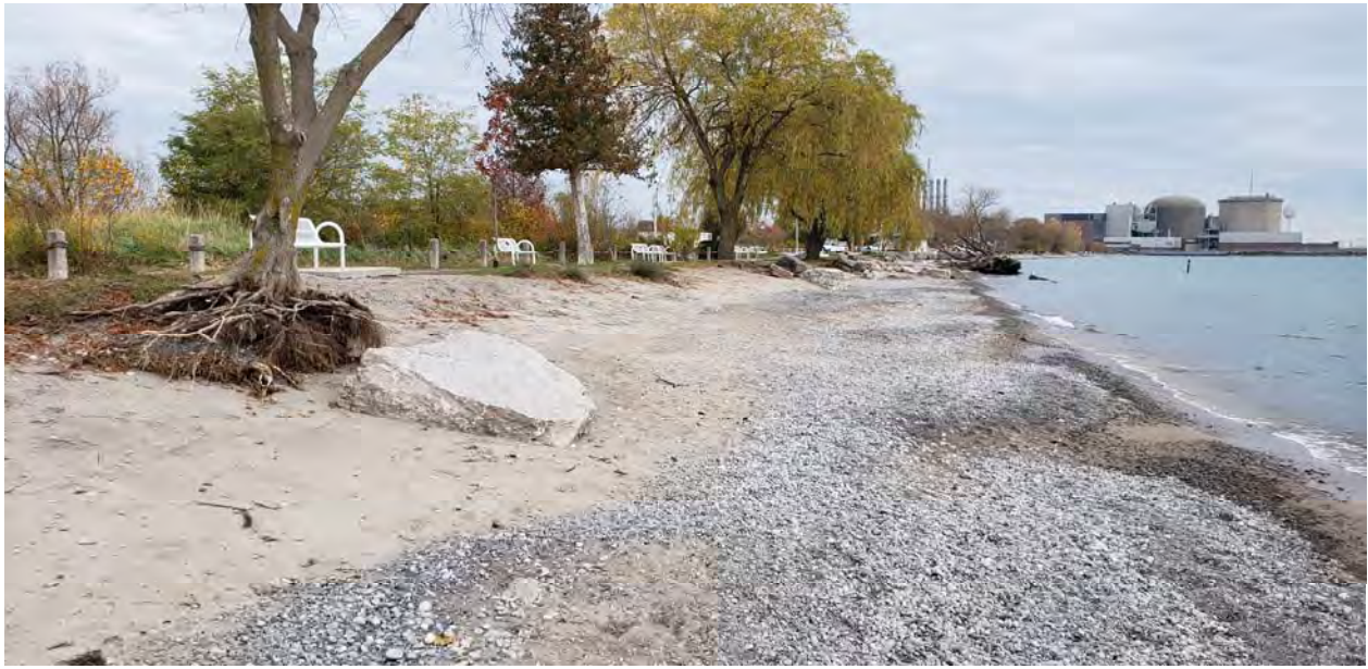
Figure 4: Beach erosion around the east end of EBB1 uprooting trees and exposing old cottage concrete stairs and foundations
