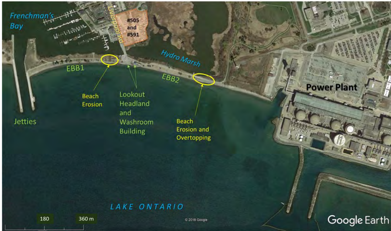
Figure 1: Overview of the project site
