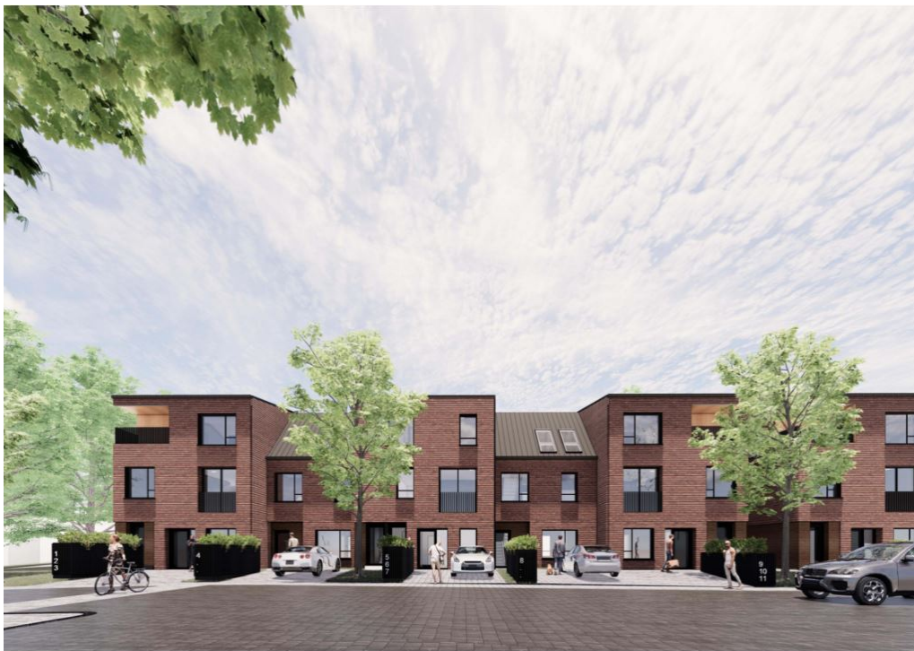
View from Internal Road
