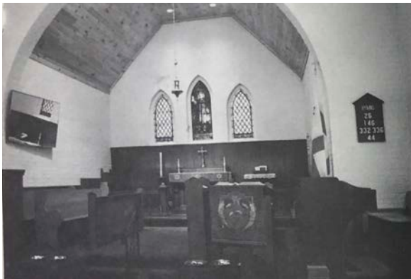
66. View to chancel after the renovation, October 1985. (St. Paul's On-The-Hill)
