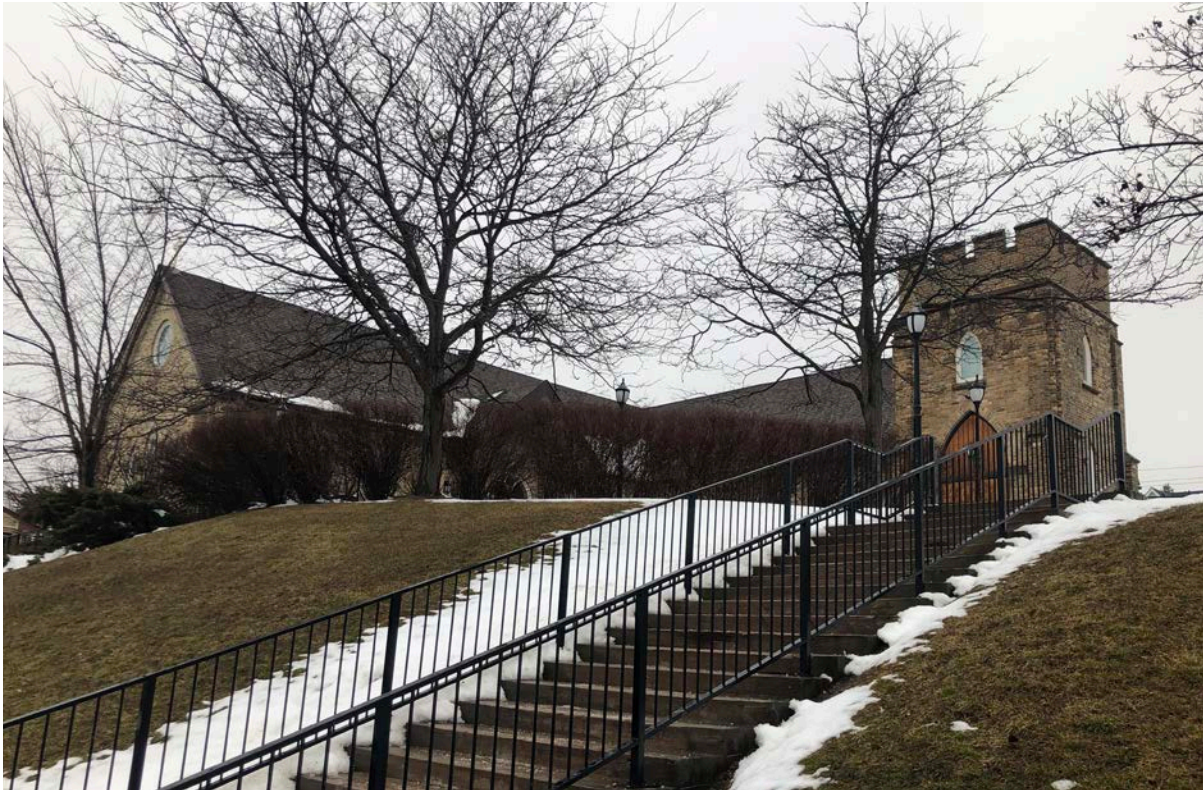
81. St. Paul's on-the-Hill as viewed from the base of the stairs at the south parking lot. (BA)
