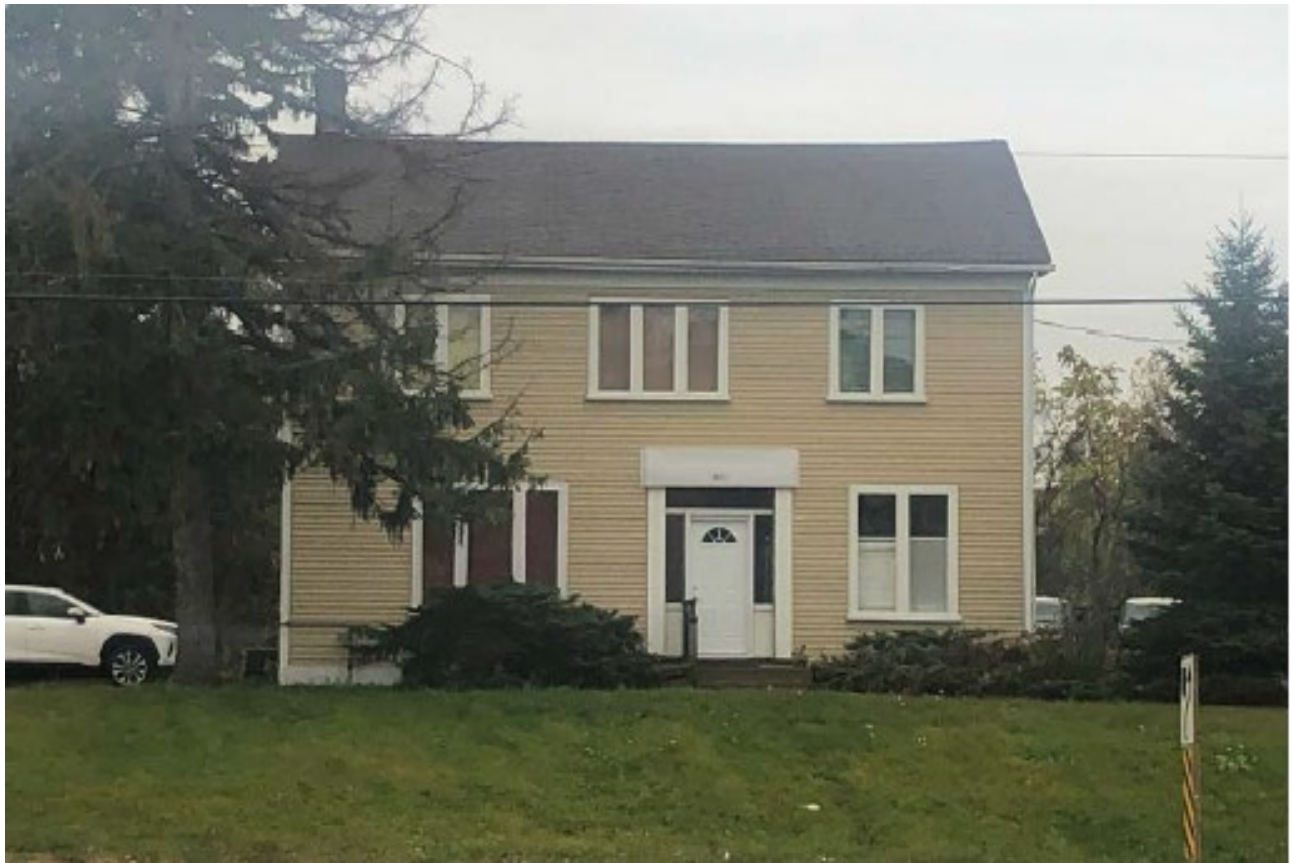
Figure 1: 301 Kingston Road, North (front) façade. Branch Architecture, 2020.
