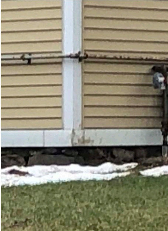
26. Stone foundation, 2019. (BA)
