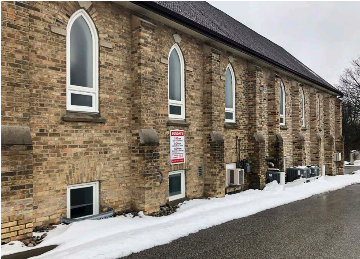
73. North elevation, original bays at left and addition at right. (BA)
