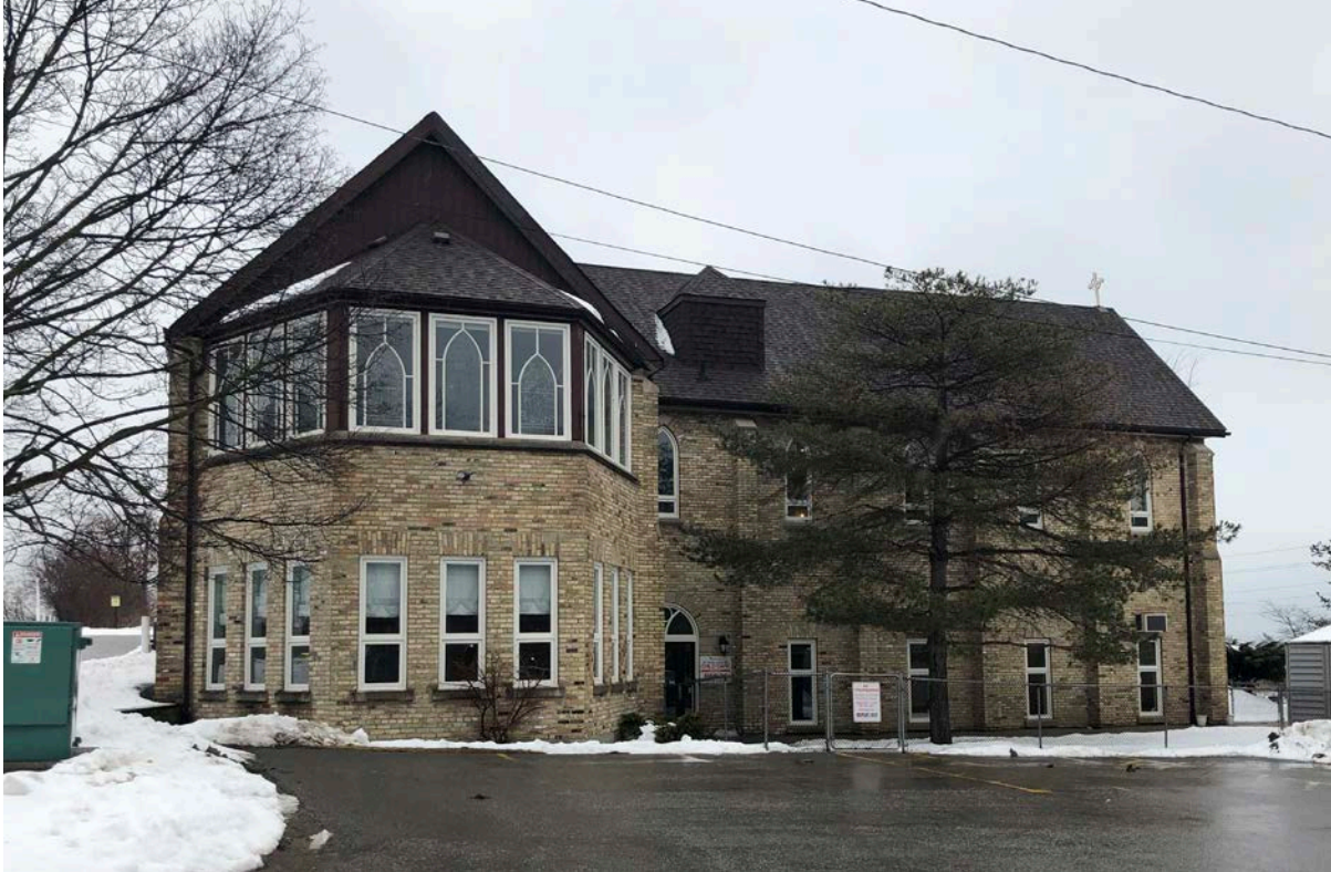
74. Addition, west elevation. (BA)
