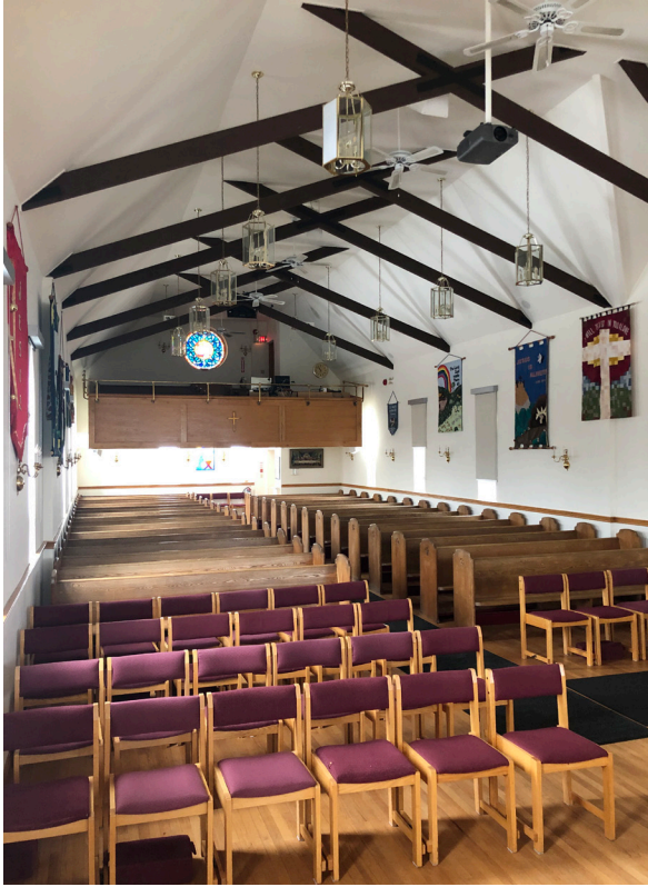
94. Nave looking to balcony. (BA)
