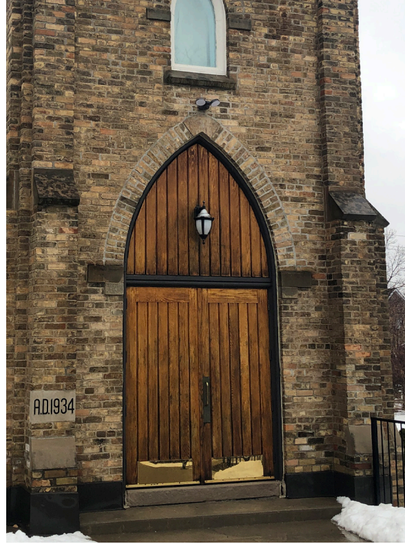
85. Original building, west entrance with 1934 date stone at left. (BA)
