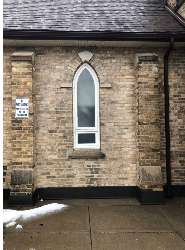
88. Original building, typical bay. (BA)
