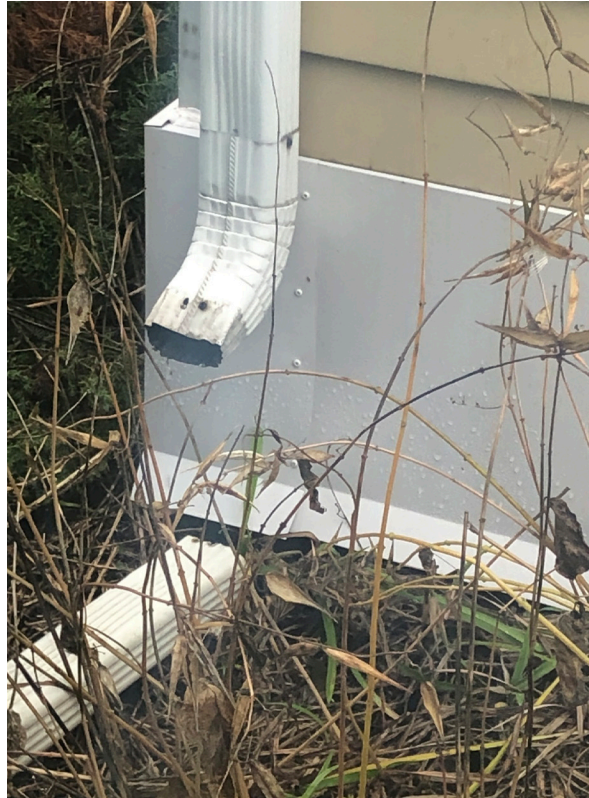
27. Metal skirt at foundation, 2020. (BA)
