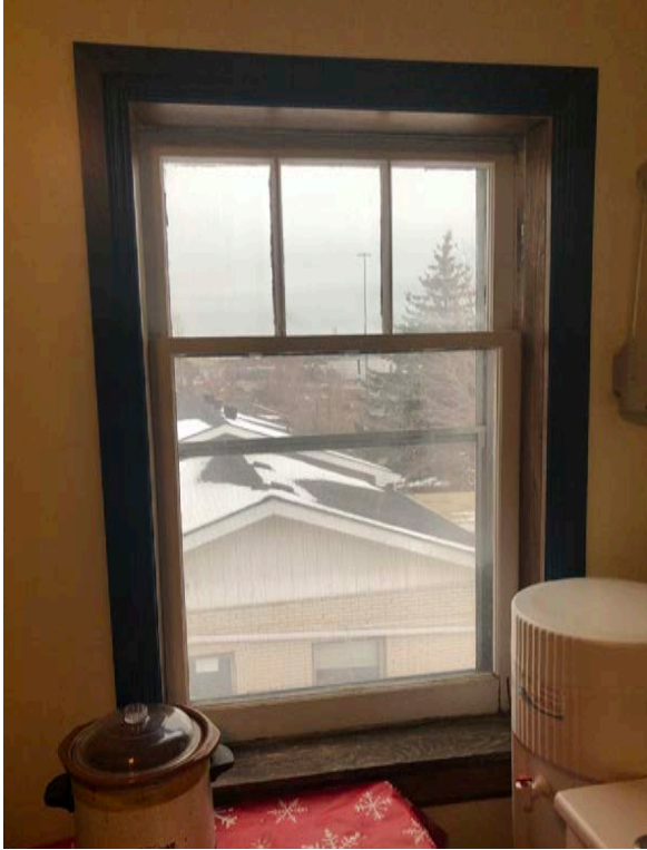
53. Interior, second floor window. (BA)
