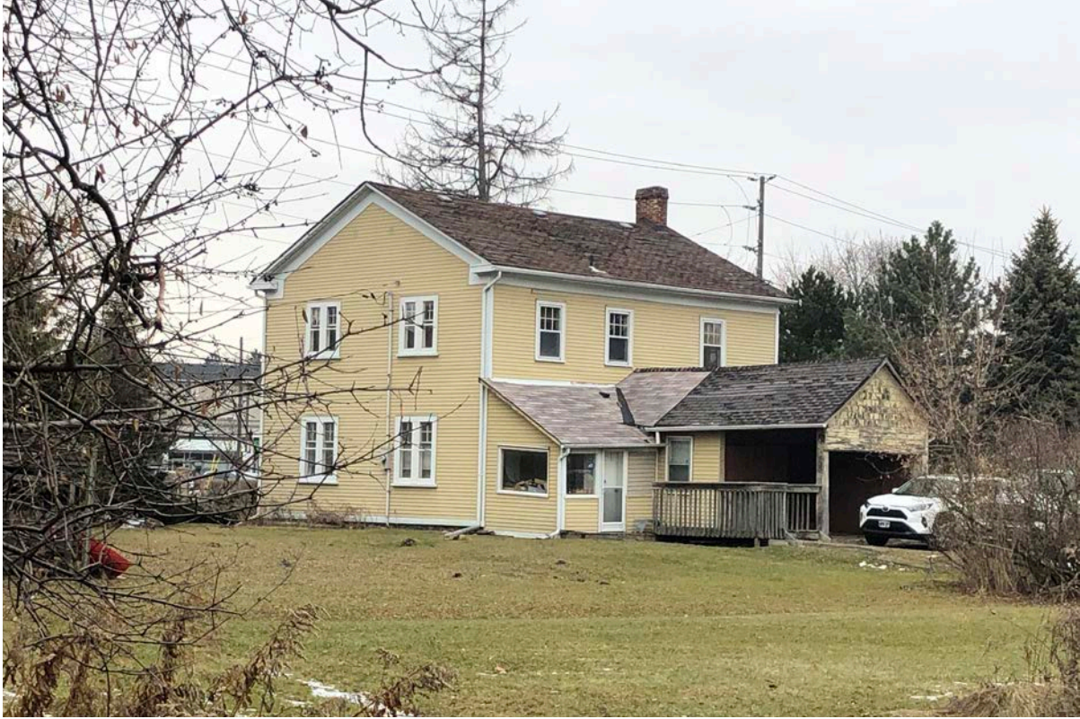
30. West (left) and south (right) elevations, 2019. (BA)
