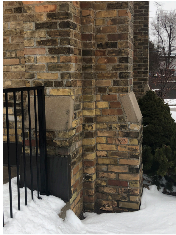
90. Original building, base of buttress with salvaged capstone. (BA)
