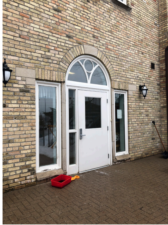
78. Addition, south entrance. (BA)
