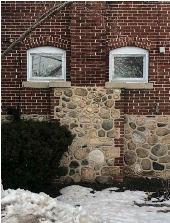
45. West elevation, base of chimney. (BA)
