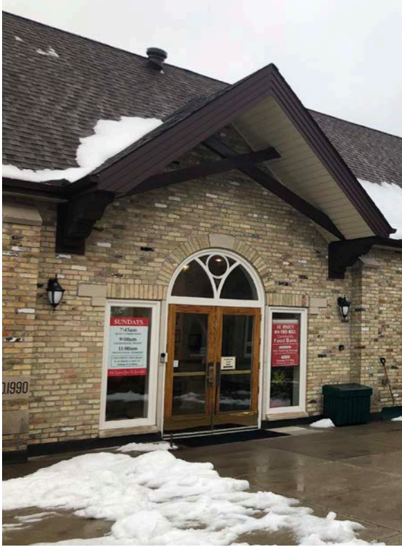
84. Addition, main entrance with 1990 date stone at left. (BA)
