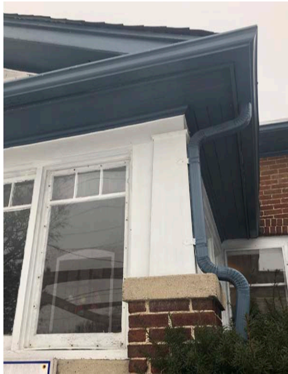
39. Porch, upper post and eaves. (BA)
