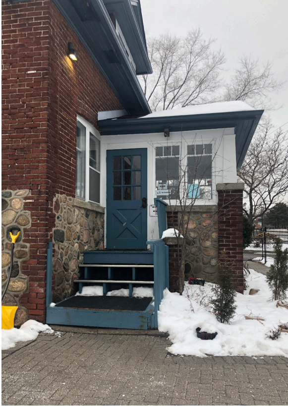
36. Porch, west elevation with entry door. (BA)
