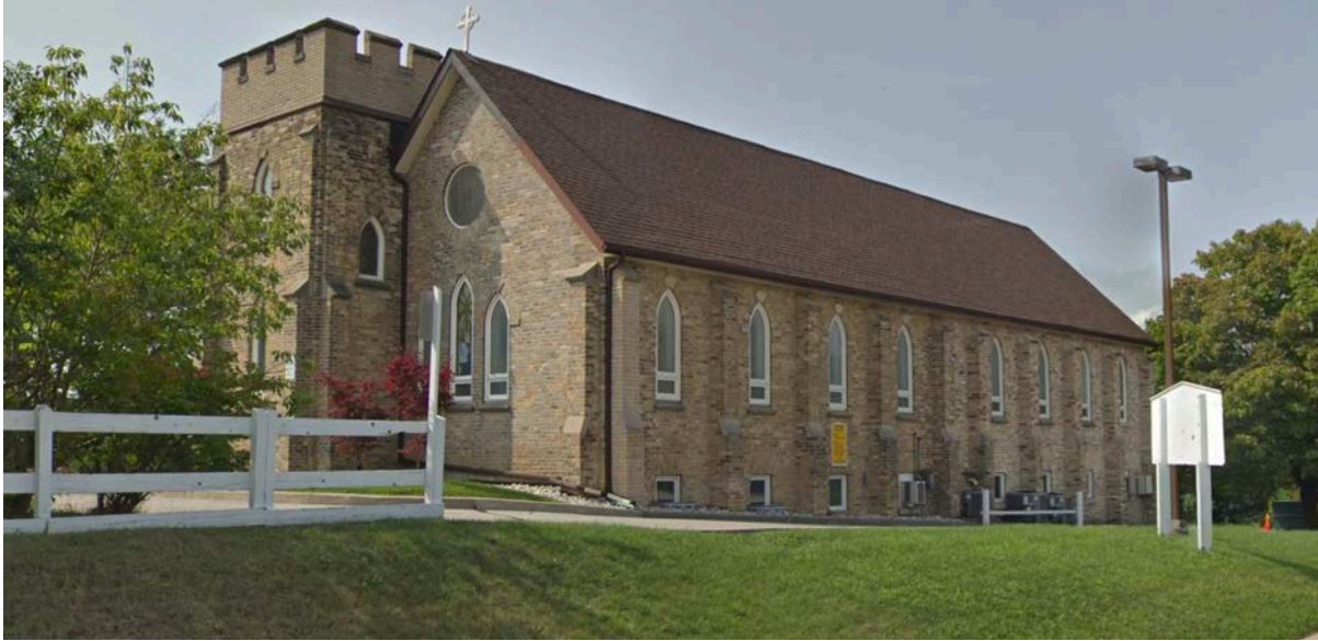
72. North elevation as viewed from Sheppard Avenue. (Google streetview)
