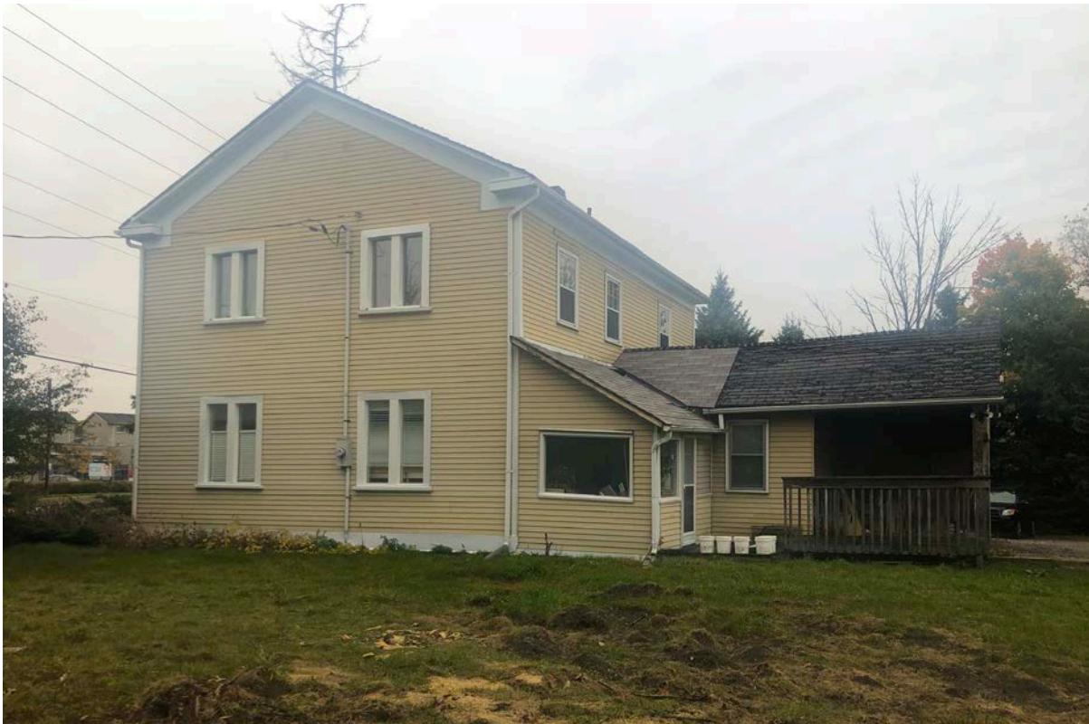
31. West (left) and south (right) elevations, 2020. (BA)
