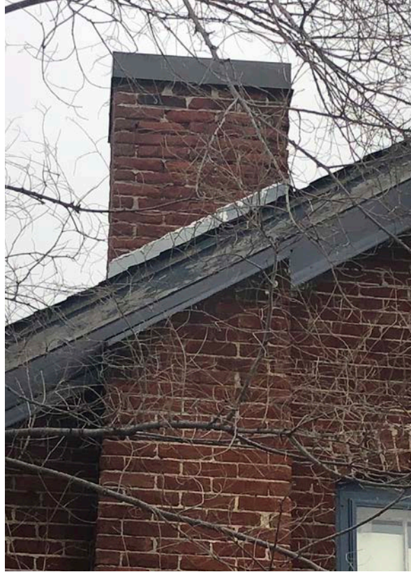
44. West elevation, chimney and eaves. (BA)
