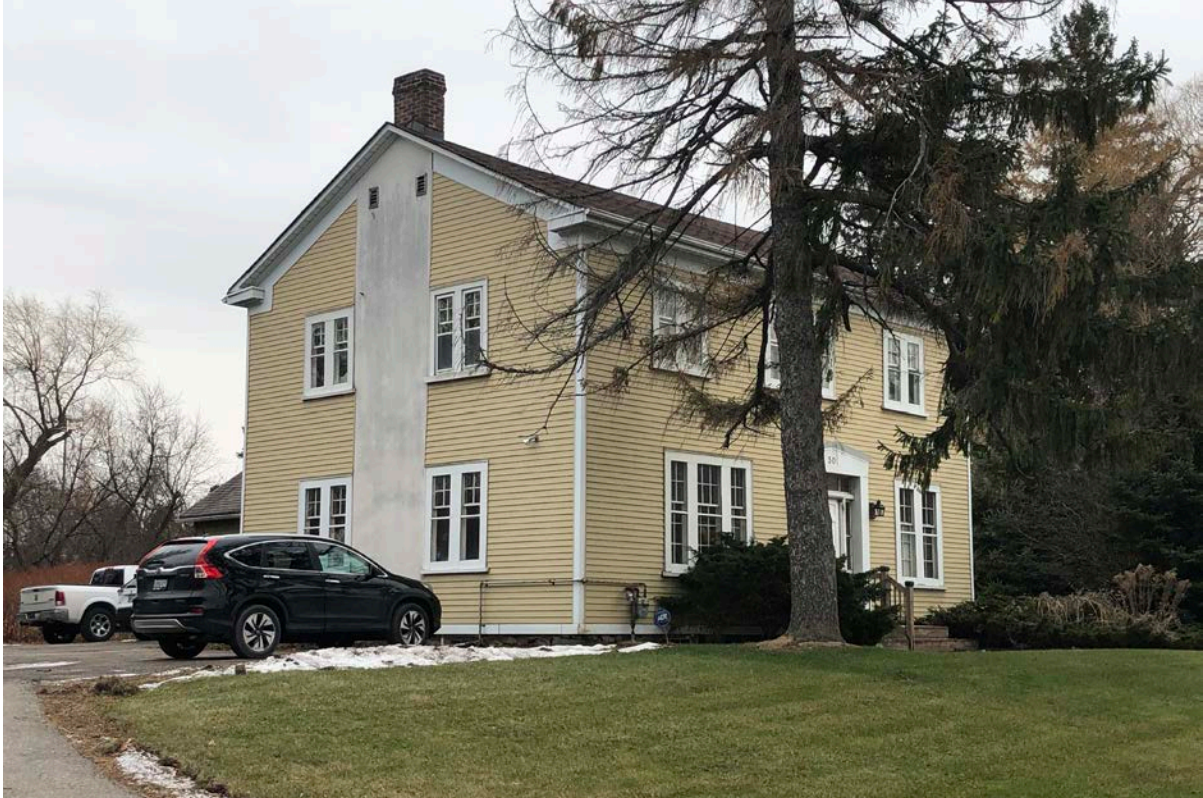
28. East (left) and north (right) elevations, 2019. (BA)
