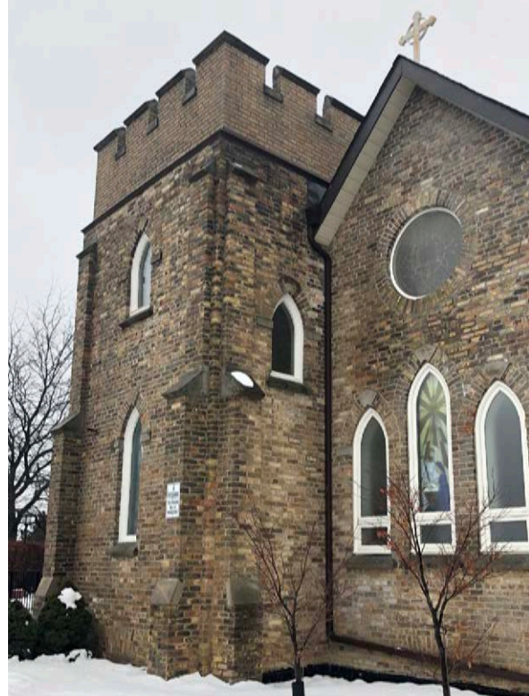
92. Original tower, east and north elevations. (BA)
