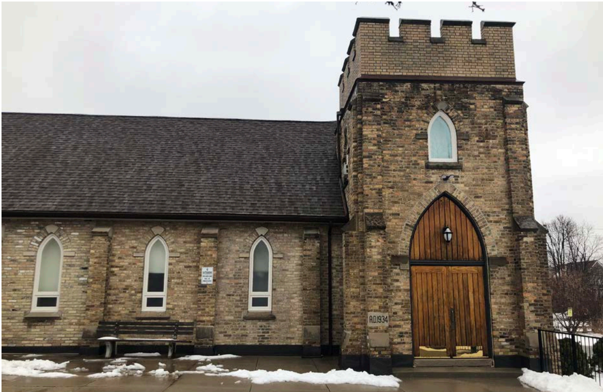
86. Original building, south elevation. (BA)
