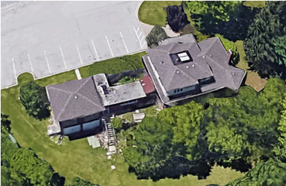
15. 1 Evelyn Avenue property, aerial view looking west, Aug. 2020. (Google streetview)
