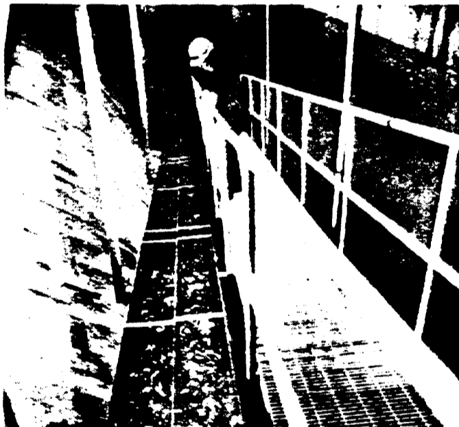
An Ontario Hydro technician looks on as thousands of American eels climb an "eel ladder" at the Robert H. Saunders - St. Lawrence Generating Station in Cornwall. The ladder was installed to allow the migrating eels to navigate the 28-metre variance in water height between the St. Lawrence River and Lake Ontario.
