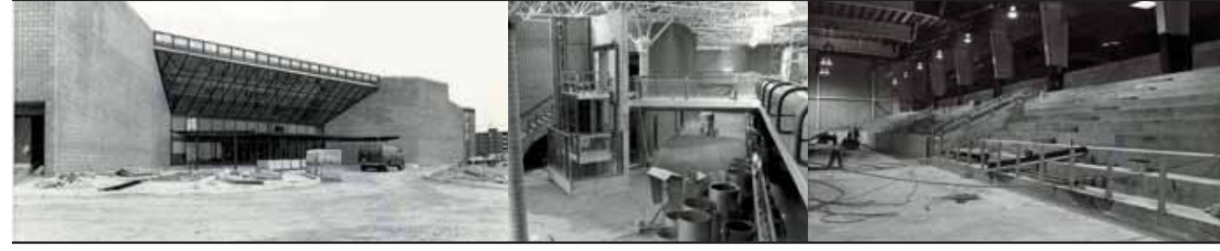
Construction of Pickering Rec Complex 1982
