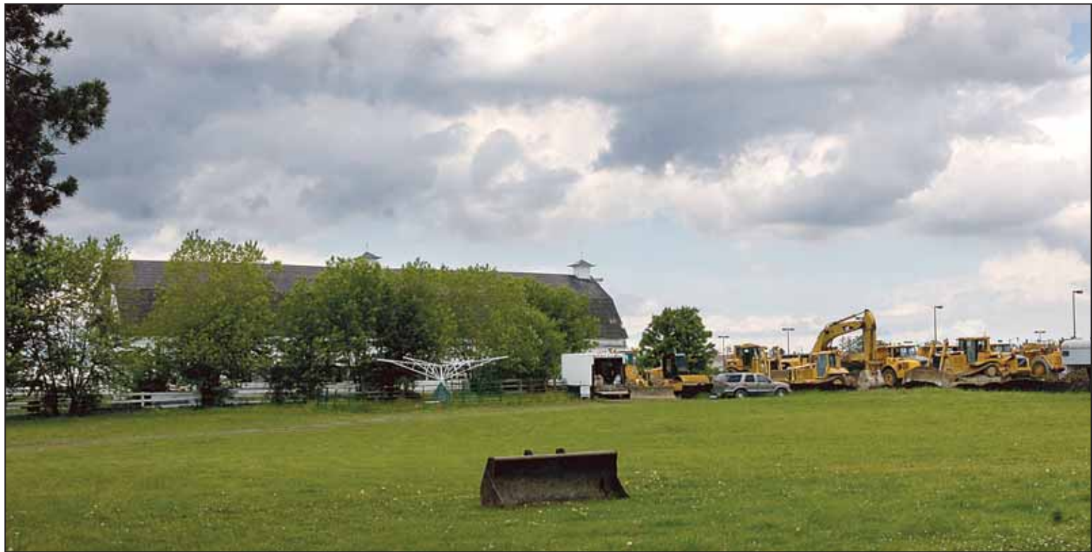
Construction vehicles sit at the ready at Picov Downs. The track's owners are planning to redevelop the track at Ajax Downs. Ron Pietroniro/ News Advertiser photo
