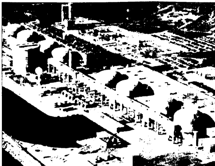
The laid up 'A' side of the Pickering Nuclear Generating Station ordered last August by Ontario Hydro's board of directors means employees at the plant are undertaking a massive shutdown operation. Taking the 'A' units off-line took four days, but they won't be in their final 'lay-up' state until the end of this month.
