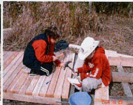
Michael and Matthew hammering boards on the board walk.
