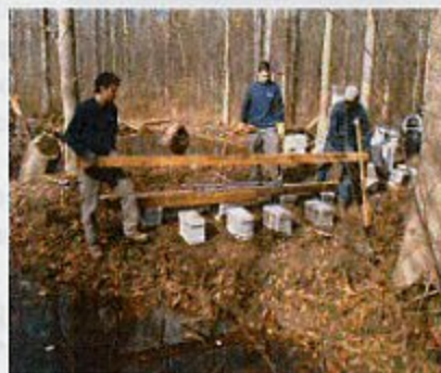
Day 24, Oct. 17, 2008 Deck constructions.
