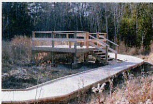
Observation deck and completed board walk.
