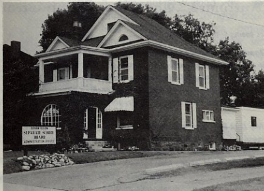
Original Board Office (1969-1982), 209 Simcoe Street South, Oshawa
