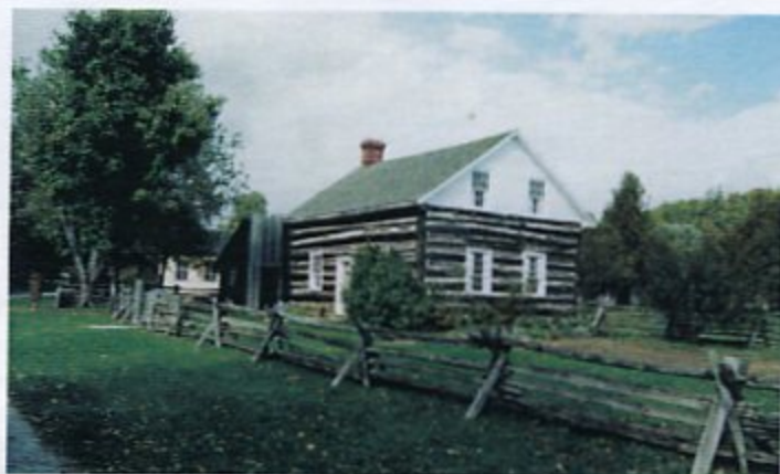
Log house at Lang Pioneer Village.
