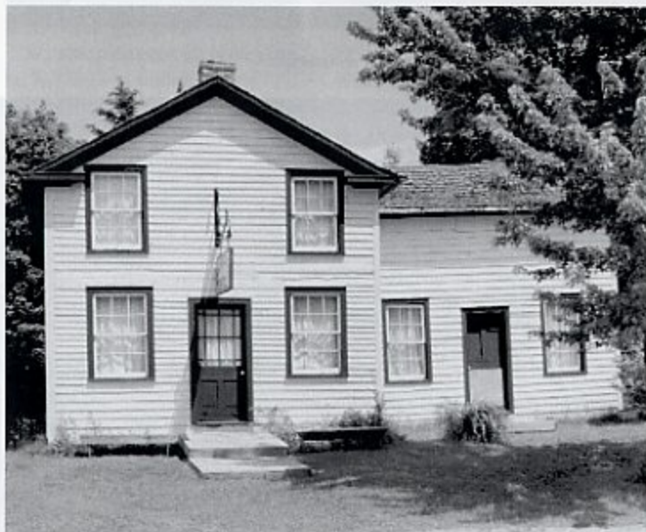
The Brougham Central Hotel as it appears in the Pickering Museum Village
