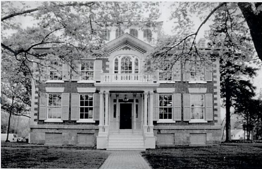
Bentley-Gibson House in 2002, just after restoration
