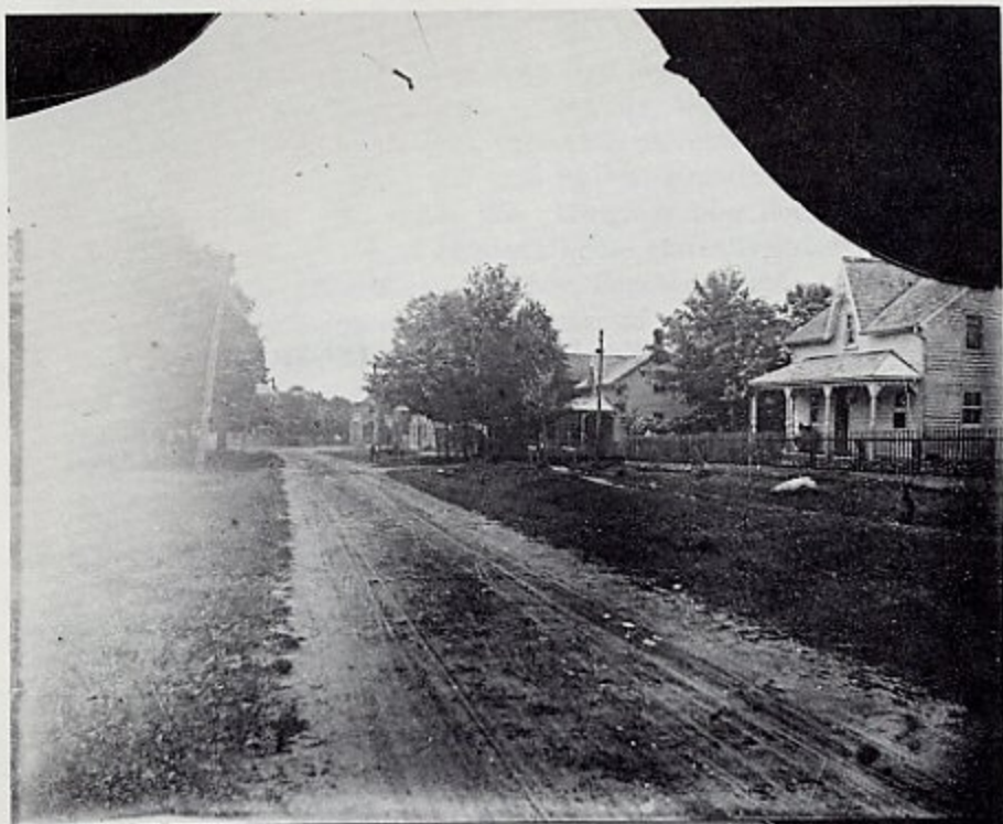
Brock Road facing South to Main Street of Brougham, Circa 1900
